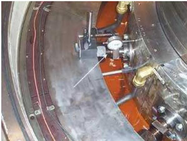
Measurements of diametrical clearance (see arrow) on the generator guide bearing on a unit at 93-MW Thompson Falls revealed the clearance had doubled over seven years of operation. Adjusting the bearing back to the original clearance solved a problem with extreme vibration.
